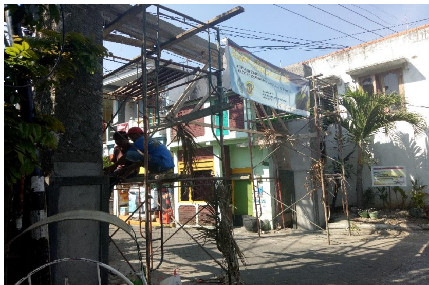
Gambar 4.5 Monitoring finishing kolom
