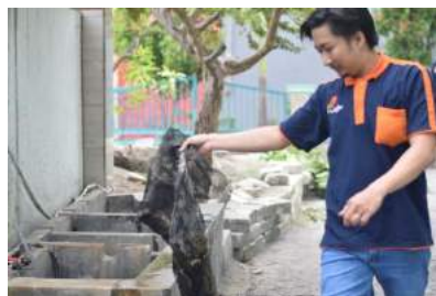
GAMBAR 7 PENCUCIAN FILTER
